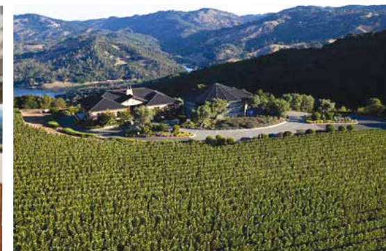
Colgin Cellars Winery
